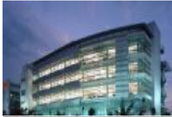
Quill Building 1 - DHL 1(c)
