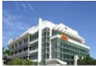
Quill Building 4 - DHL 2(c)
